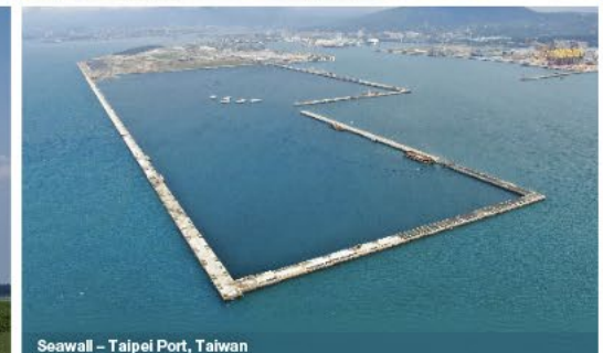
Seawall - Taipei Port, Taiwan
