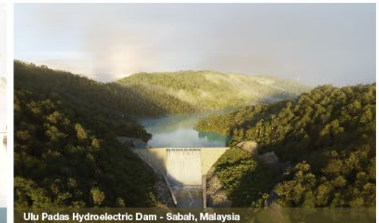
Ulu Padas Hydroelectric Dam - Sabah, Malaysia
