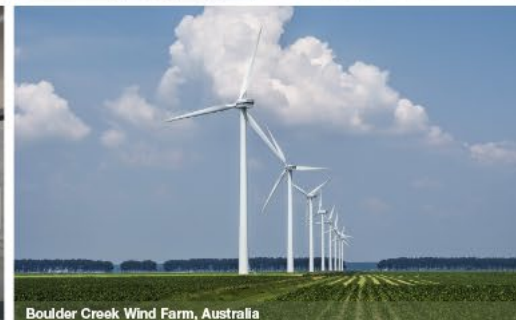
Boulder Creek Wind Farm, Australia
