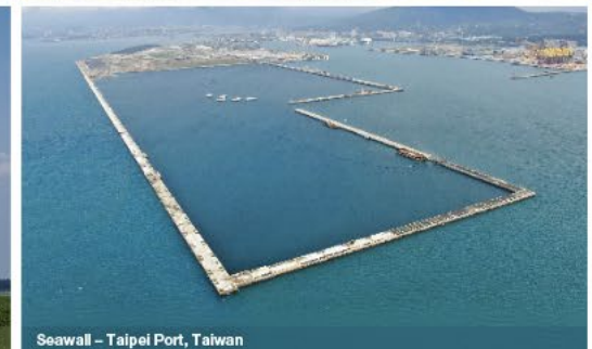
Seawall - Taipei Port, Taiwan
