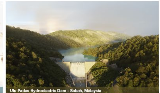
Ulu Padas Hydroelectric Dam - Sabah, Malaysia
