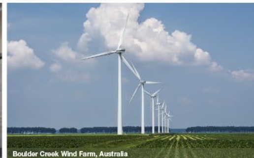
Boulder Creek Wind Farm, Australia
