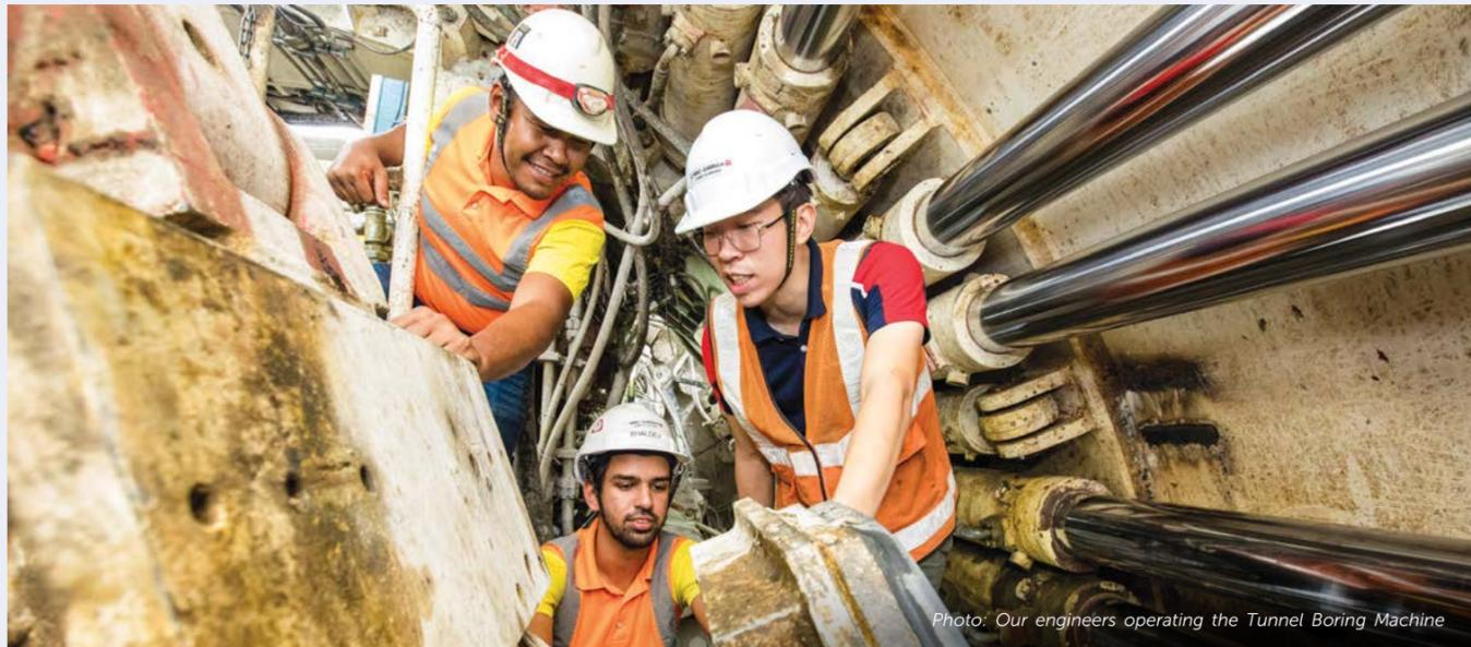
Photo: Our engineers operating the Tunnel Boring Machine
