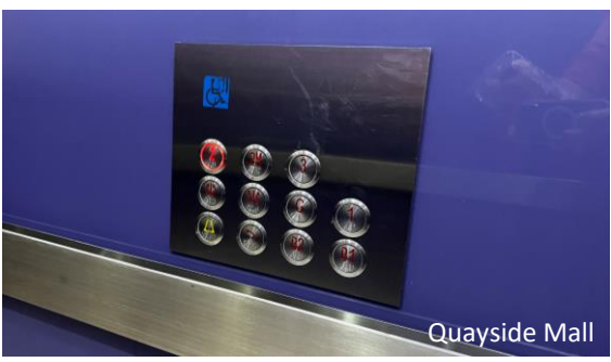
Elevator button with the braille feature and positioned at waist-level
